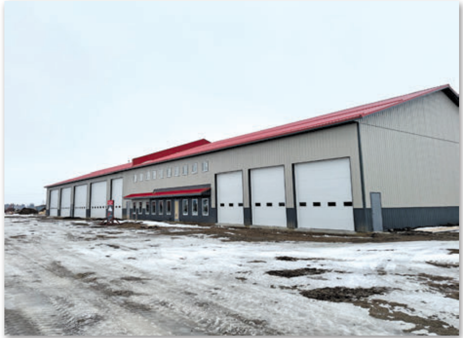
The new Martodam Motors facility, located on the north side of Highway 3, is almost ready for move-in day.
