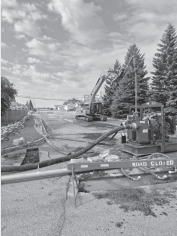
An unexpected storm sewer issue on 1st Street East in Shellbrook had crews on site dewatering the area much of last week.
