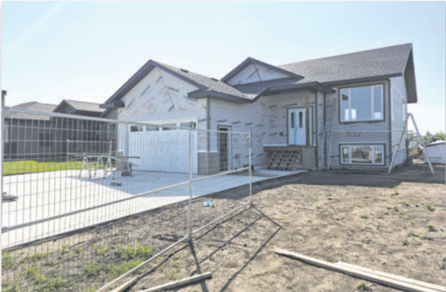
The Shellbrook and District Health Foundation is currently building housing for healthcare professionals in Shellbrook.
