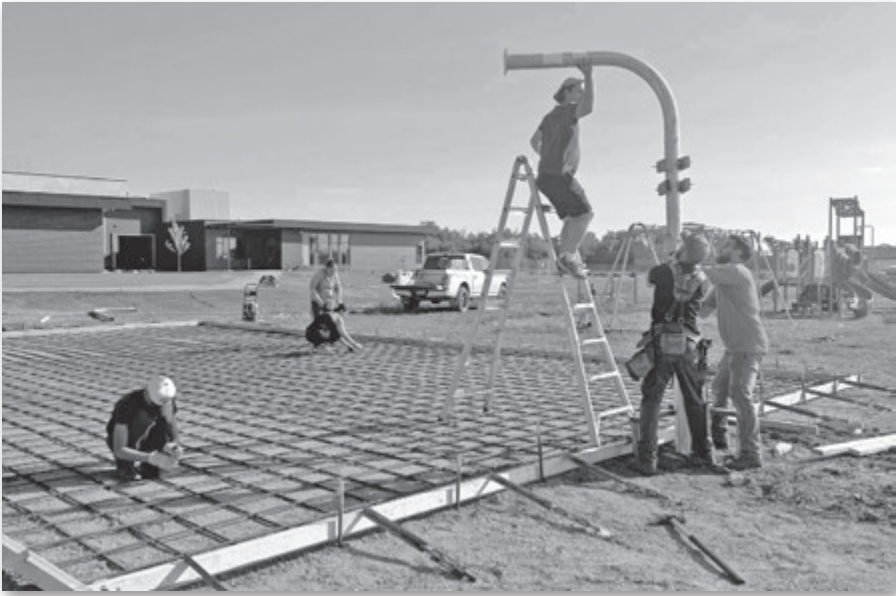
Crews work on the frame for the concrete and set up the pools for the hoops.
